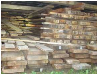
Detail of stacked Coach House components showing organization and tags. (ERA, 2017)
