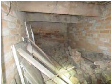
Interior of central crawlspace under rear kitchen addition. (ERA, 2017).
