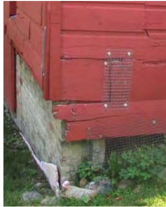
Left: South elevation of rear kitchen addition Right: Detail of rebuilt west foundation wall that does not return at south. (ERA, 2017)
