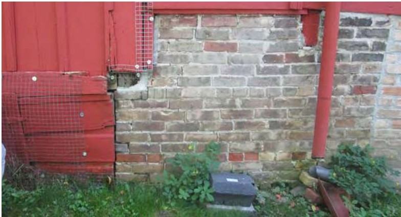
Brick Foundation Wall at north portion of west elevation of kitchen addition. (ERA, 2017)
