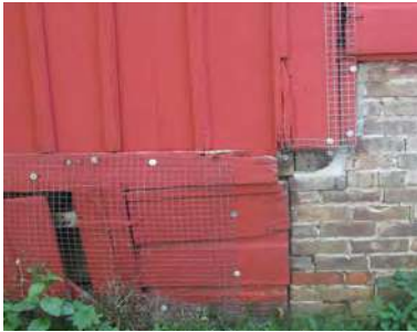
Area for review and repair of wire mesh at rear kitchen addition. (ERA, 2017).
