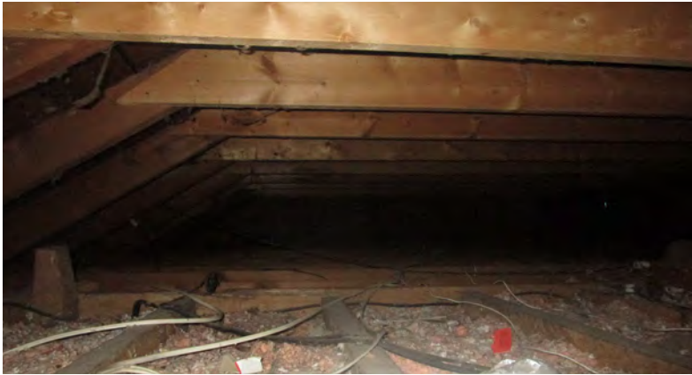
Interior of eastern (main house) attic, with tie reinforcement, wiring, and blown in insulation shown. (ERA, 2017).
