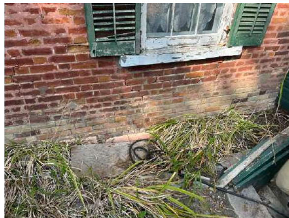
Foundation at South elevation of ball room, closed-off crawlspace venting.
