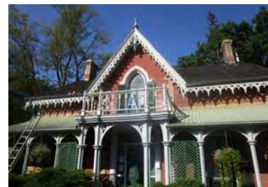
East Elevation (ERA, 2017).
