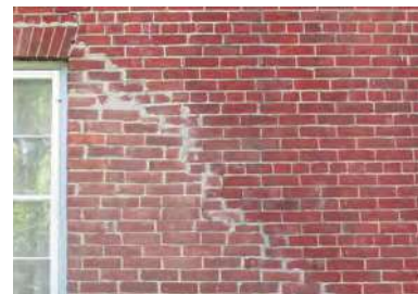
Portland cement repair of step crack-ing at north elevation (ERA, 2017).
