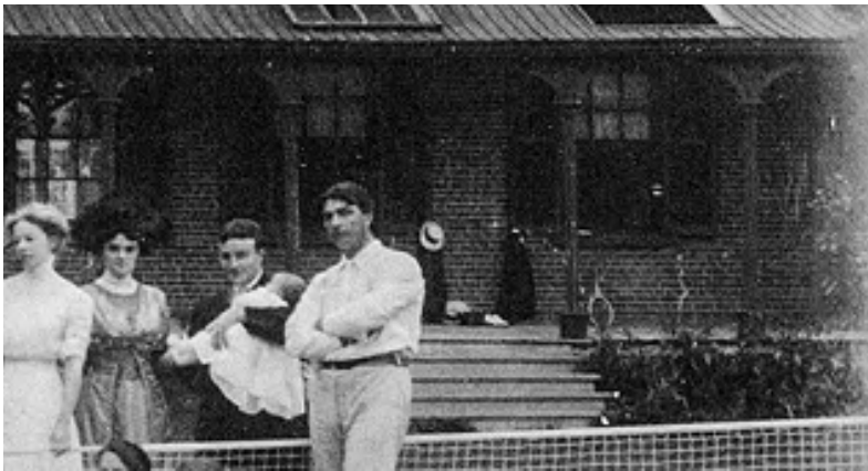
Excerpt of archival photograph showing north veranda staircase position and style. (AHS)
