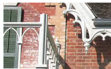
Brick masonry at the east elevation (ERA, 2017).
