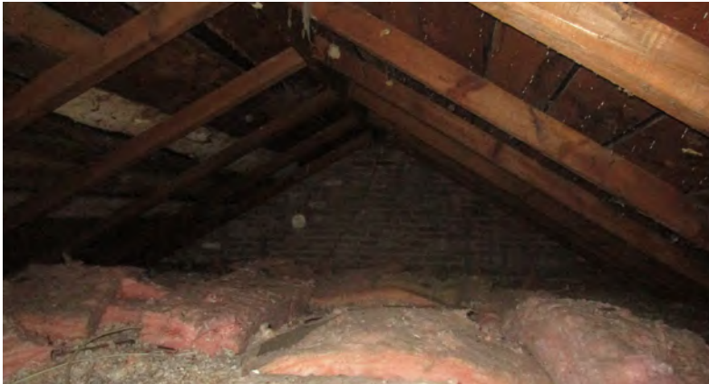
Interior of western (1869 addition) attic, showing framing, and multiple layers of insulation. (ERA, 2017)
