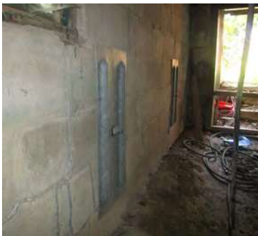
Steel plates installed to reinforce block wall under south veranda. (ERA, 2017).
