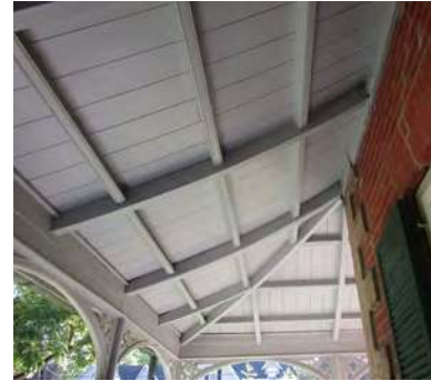
Porch soffit, Hillary House. (ERA, 2017)
