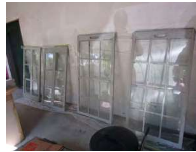
Window restoration at Hillary House. (ERA, 2017).
