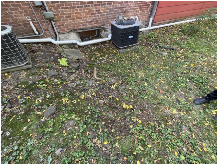
Photo 2: Adjacent grading (typical at multiple locations)
