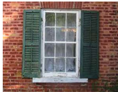
Wood window and shutters at south elevation of 1879 addition (ERA, 2017).
