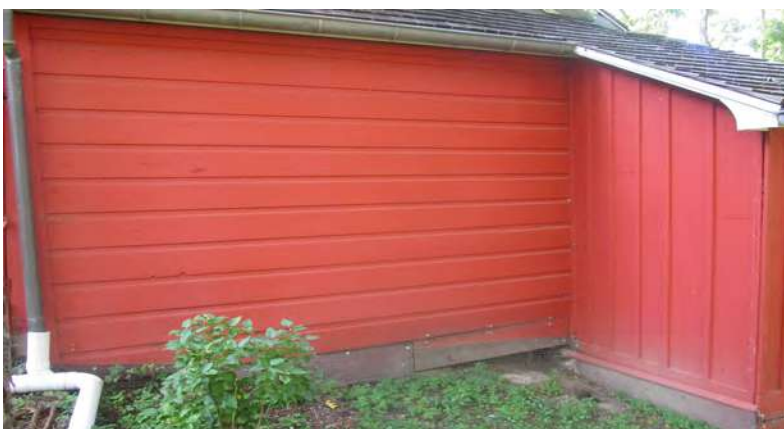
North elevation of rear kitchen addition, showing corridor and privy structures. (ERA, 2017)
