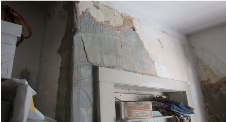
Wallpaper at second floor nursery (now storage room). (ERA, 2017)
