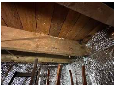
Basement waterproofing concealing masonry wall
