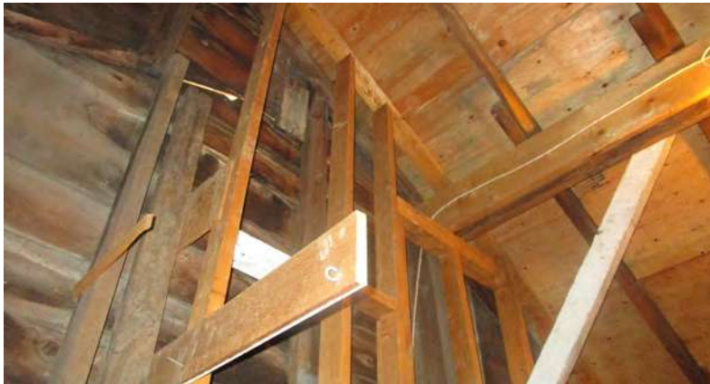
Remediation of framing at the interior of the rear summer kitchen addition. (ERA, 2017)
