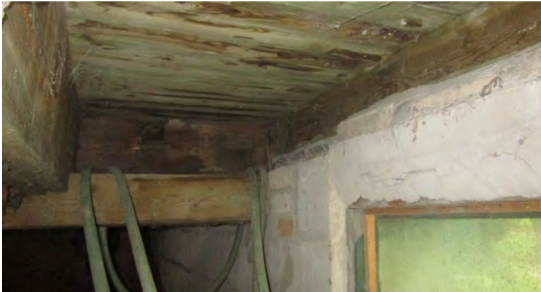
Underside of south veranda floor at area of concern, showing the wide span made by the floorboards in the area at the top of the steps. (ERA, 2017)
