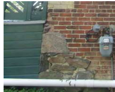
Keying of field stone and brick at base of west elevation. (ERA, 2017).
