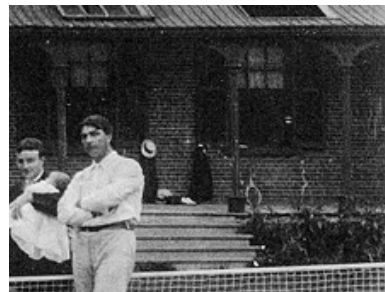
North veranda staircase to be restored. (AHS).
