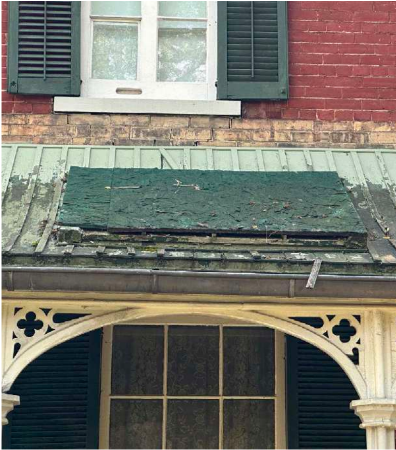
Skylights at veranda roof.
