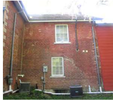
Masonry for review at North elevation of 1869 addition. (ERA, 2017).
