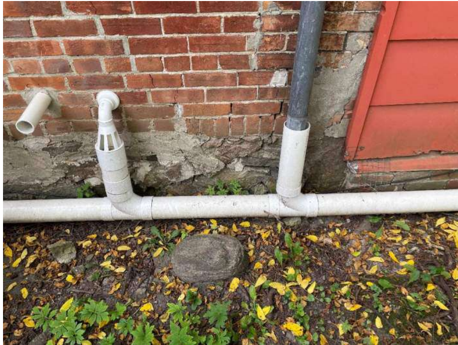
Photo 7: Phase 3 construction appears to be slab on grade.
