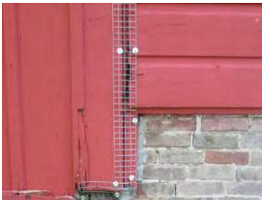
Typical repairs to building fabric to prevent entry of animals. (ERA, 2017).
