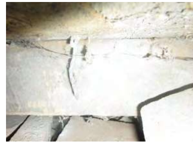
Underside of rear kitchen addition flooring, showing wood sleepers resting on irregular joist fabric. (ERA, 2017)
