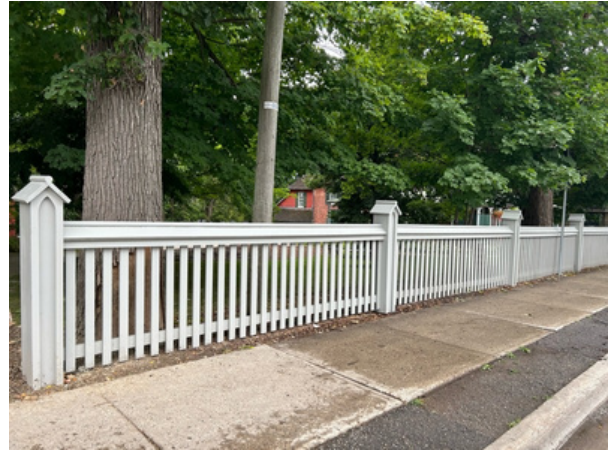
Repaired Fence, August 2024
