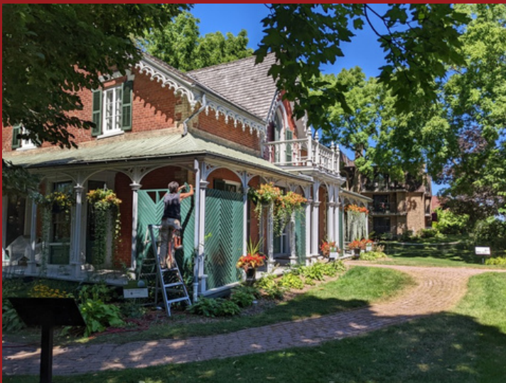
Restoration of the lattice panels.
