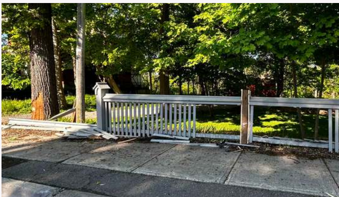
Damage to our heritage fence occurred afterhours on Thursday, May 23rd, 2024.
